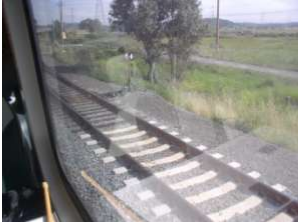
The double tracks where trains can pass.
