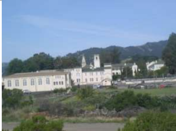
St Vincents School from the rear.
