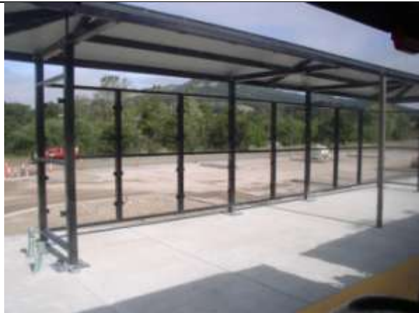
The incomplete Novato North station.
